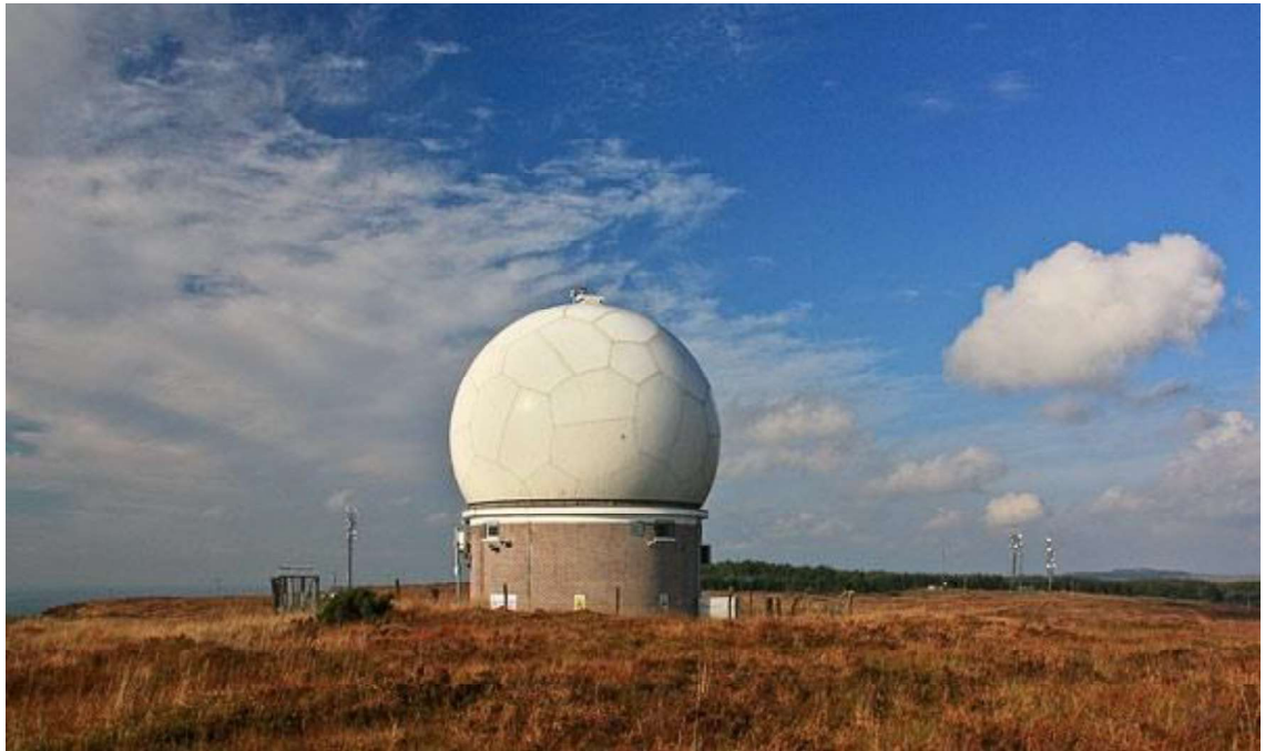
Figure 3.3 The stand-alone en-route MSSR at Woodcock Hill housed in a radome (Image source: IAA).
